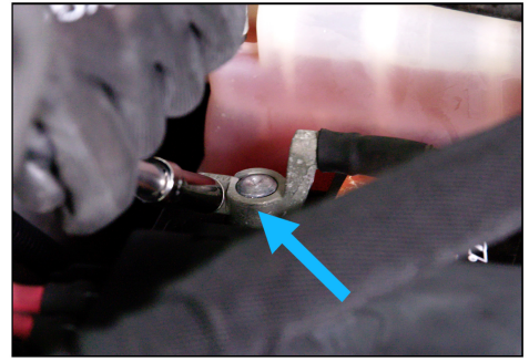
19. Reconnect the negative battery cable using the 10mm socket.
